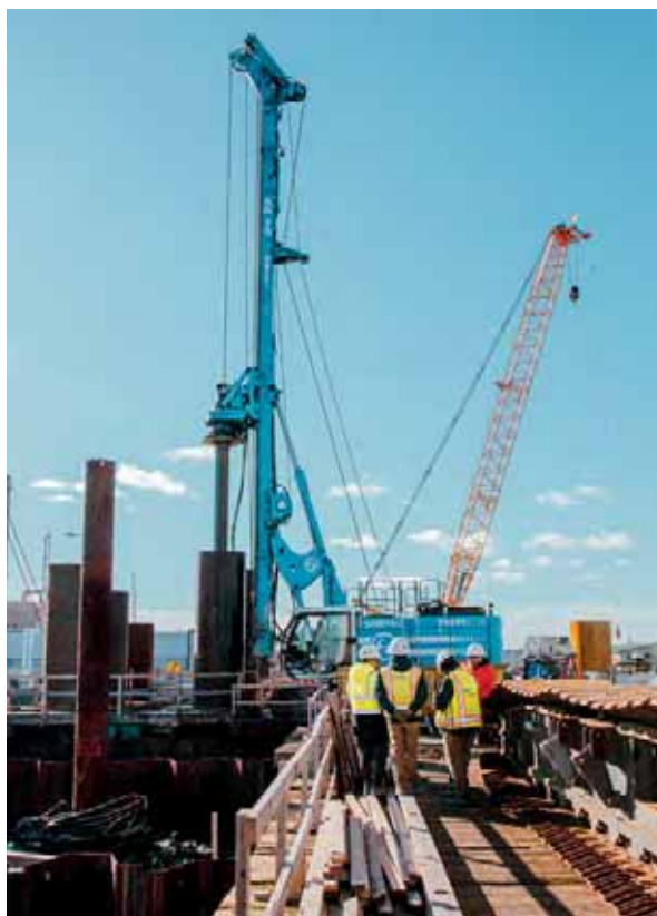
Belden Bly bridge project | MA, USA
